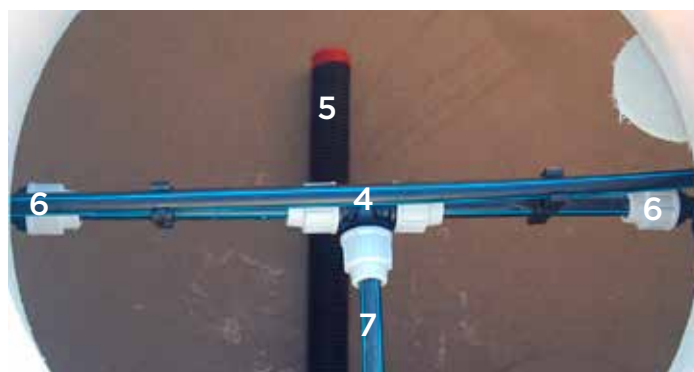
Spredesystemet i biofilteret
