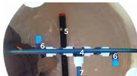
Spredesystem i stor biofilterkum
